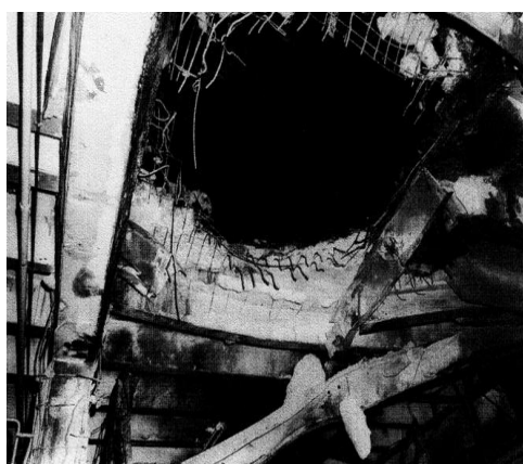
Fig. 1-1 View of the site after a thermal explosion of a reaction vessel
